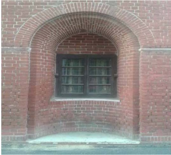
Fig. 4: Window with the deepest external shading device
